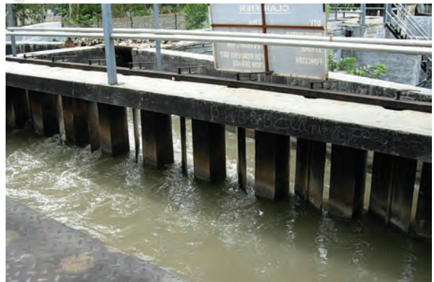
Fig. 18.4 Grit and sand removal tank
